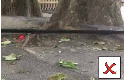
UNDULATIONS ARE GREATER THAN 10MM
