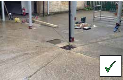
CONCRETE HAS BEEN LAID TO FALLS
