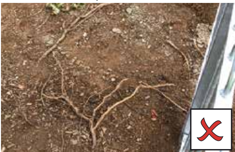
SURFACE IS NOT CLEAR OF TREE ROOTS
