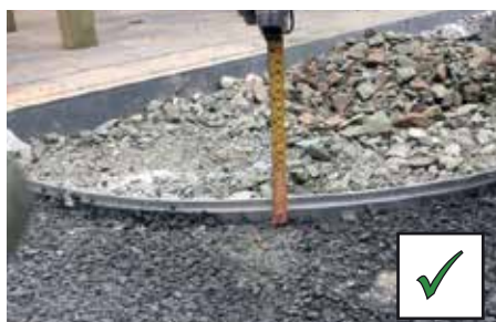
HEIGHT OF EDGE IS EQUAL TO DEPTH OF NEW SURFACE
