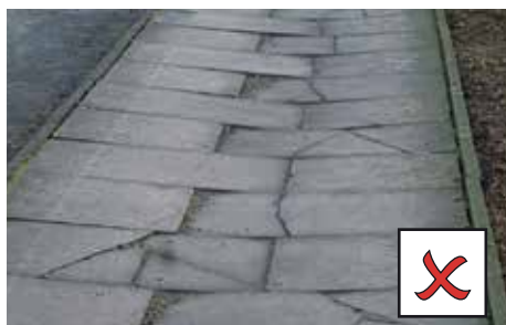
FLAGS ARE NOT FLAT, LEVEL OR CRACK FREE
