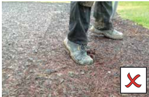
SOFT SPOTS CAN BE CREATED WHEN MULCH IS LAID ONTO WET SOIL / GRASS
