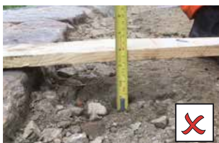
HEIGHT OF EDGE IS NOT EQUAL TO DEPTH OF NEW SURFACE
