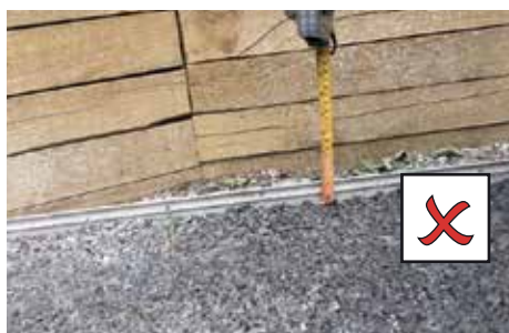
HEIGHT OF EDGE IS NOT EQUAL TO DEPTH OF NEW SURFACE
