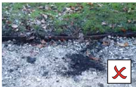
EDGES ARE NOT STRAIGHT OR CLEAN. THIS PREVENTS A STRONG BOND WITH THE EDGE
