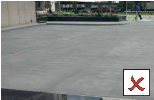
CONCRETE HAS NOT BEEN LAID TO FALLS
