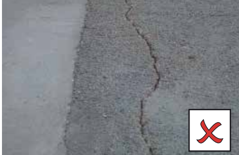
SURFACE IS NOT OF SOUND CONSTRUCTION
