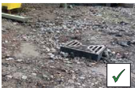
A DRAINAGE GULLY HAS BEEN INSTALLED. MOT STILL TO BE COMPLETED
