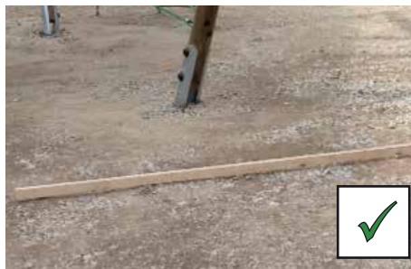
UNDULATIONS ARE LESS THAN 10MM
