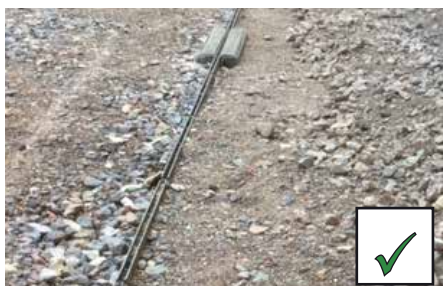
A DRAINAGE CHANNEL HAS BEEN INSTALLED. MOT STILL TO BE LEVELED
