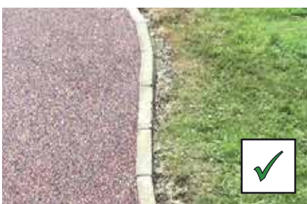
NEW SURFACE IS FLUSH WITH EDGE
