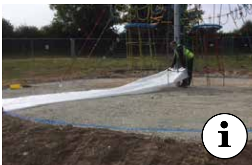
GEOTEXTILE LAYER LAID IN ADVANCE TO PREVENT WEED GROWTH
