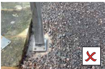
HOLES HAVE NOT BEEN BACKFILLED
