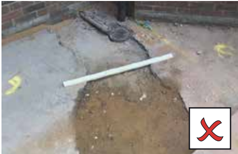
CONCRETE BASE IS NOT LEVEL
