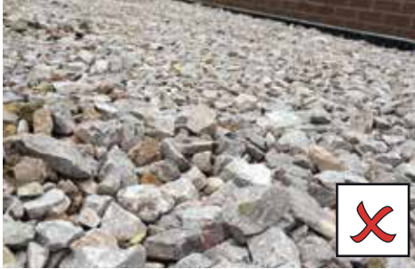
SUB BASE CONTAINS LARGE STONES WITH NO FINES
