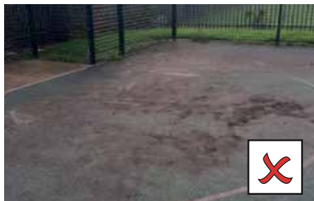
SURFACE IS CLOGGED WITH DIRT - AREA IS NO LONGER PERMEABLE
