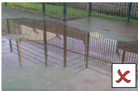
SURFACE IS CLOGGED WITH DIRT - AREA IS NO LONGER PERMEABLE
