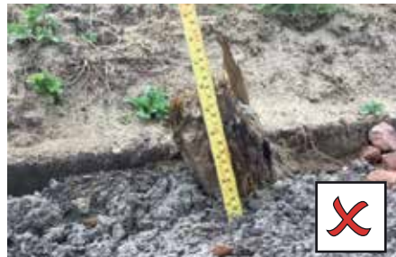
WETPOUR CANNOT BE INSTALLED DIRECTLY TO THE EDGE
