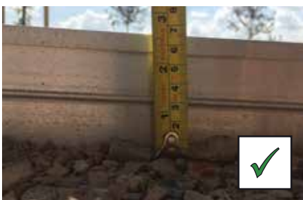
HEIGHT OF EDGE IS EQUAL TO DEPTH OF NEW SURFACE
