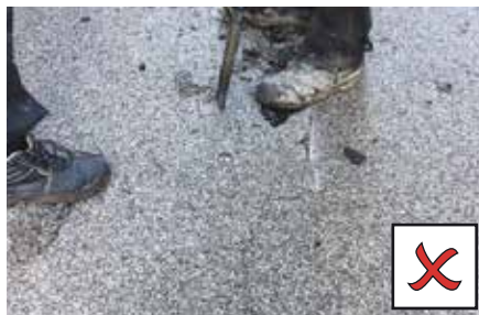
REFLECTIVE CRACKING FROM MACADAM SUB-BASE
