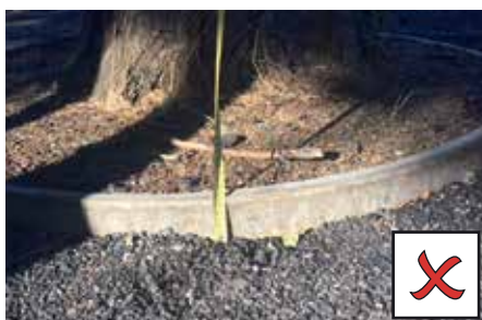
SOME SECTIONS OF EDGES ARE NOT LEVEL
