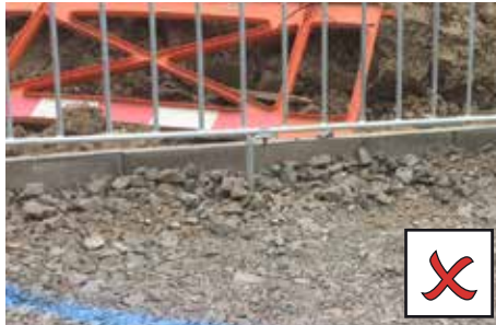
EDGES REQUIRE COMPACTING
