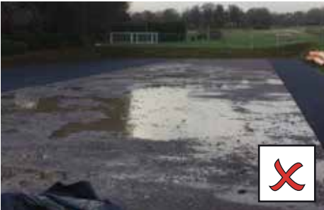
SUB-BASE IS NOT SOLID OR COMPACT - NEEDS TO DRY BEFORE INSTALL
