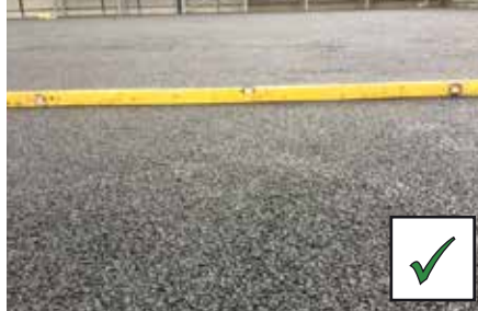
UNDULATIONS ARE LESS THAN 10MM
