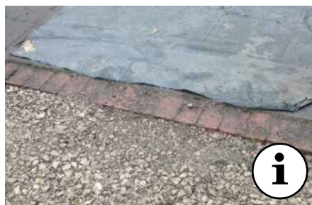
EDGINGS ARE NOT EQUAL TO THE DEPTH OF THE NEW WETPOUR SURFACING - RAMP DOWN REQUIRED
