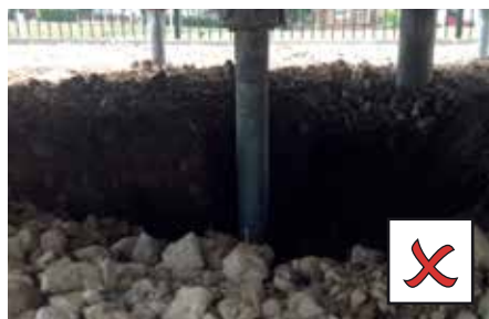
SURFACE IS NOT LEVEL UNDER EQUIPMENT
