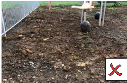
TEXTURE OF SOIL IS INCONSISTENT
